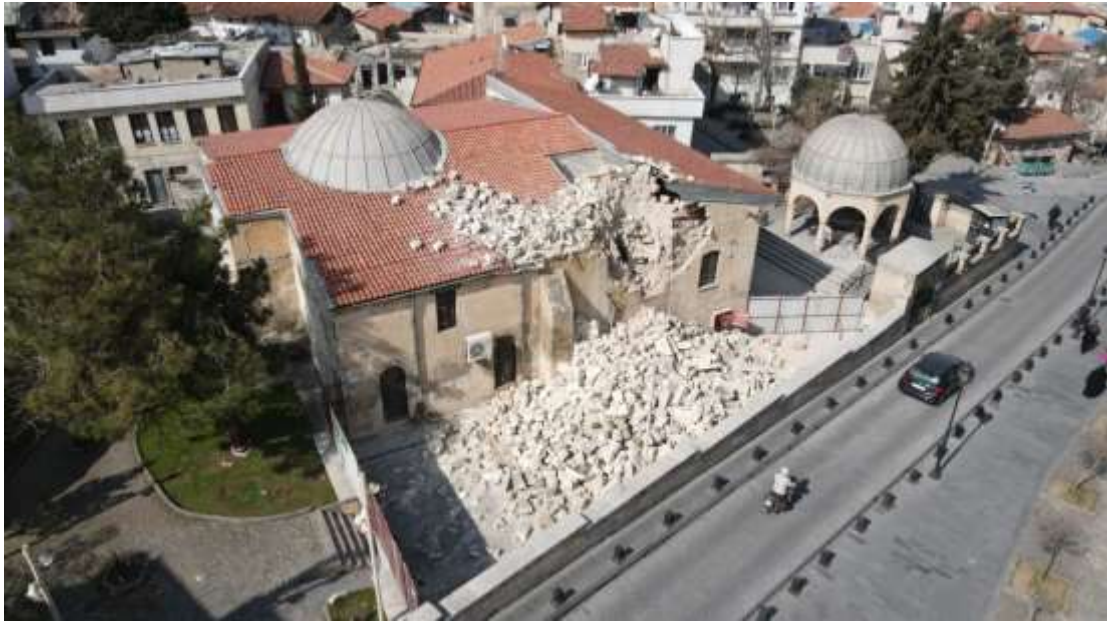
Fig. 2 The Minaret of Şirvani Mosque after the earthquake
