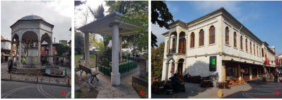
Figure 7. Images of Şadırvan (a), Ebu Derda Hz. Tomb (b) and Old Municipality Building (c) (Original, 2018)
