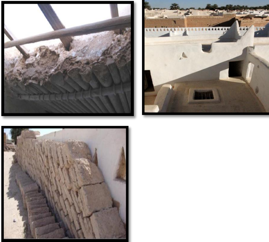
Figure 8. The roofing is constructed using palm trunks, and the will used clay bricks and small stone. (Shahran 2018)
