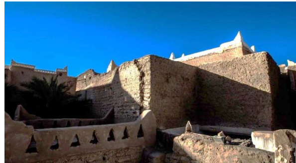
Fig: 15 The contiguity of houses minimizes the exposure to sun. Image source from Google earth, (2022)
