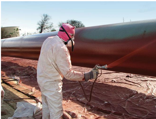
Figure 2: Application of Water based corrosion inhibition on pipeline
