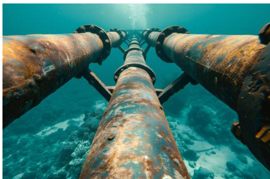
Figure 1: rusting of pipelines in the sea
