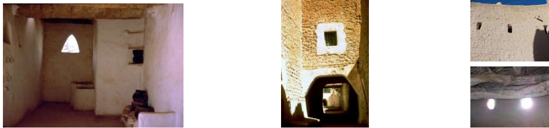
Fig: 12 Small openings on the walls and roof of the courtyard (Alhamali Y, 2013)
